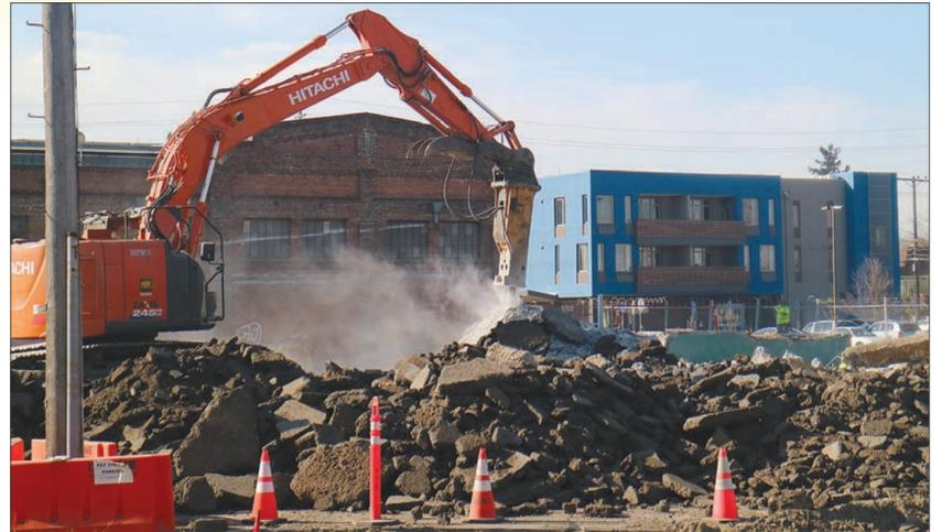
An excavator with a hydraulic breaker goes to work on concrete remnants outside the Del Monte warehouse on Buena Vista Avenue.
